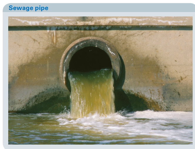
Fig. 1: Outflow pipe for wastewater containing sludge - a nightmare for analytical chemists
